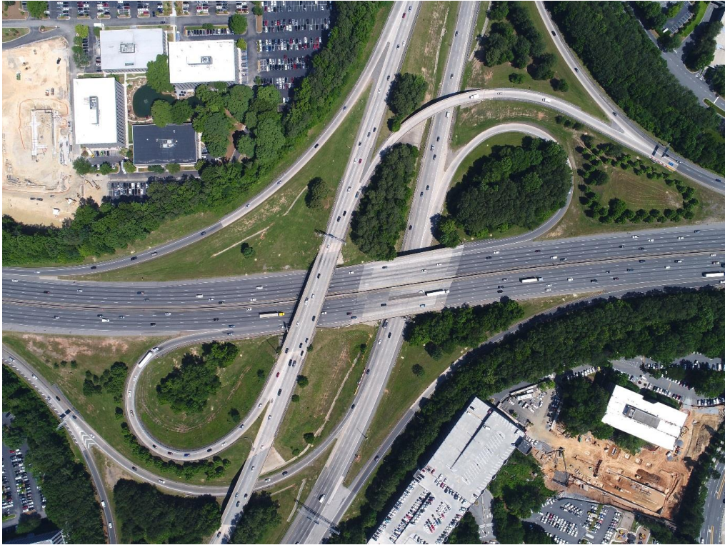
Former Interchange Prior to start of construction
